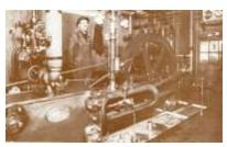
Recent New Glarus community meetings are drawing attention to New Glarus Power and Light and water services. New Glarus has had its own Power and Light Company since 1902. At that time, the power came from a 30-horsepower double cylinder gas engine. The plant
