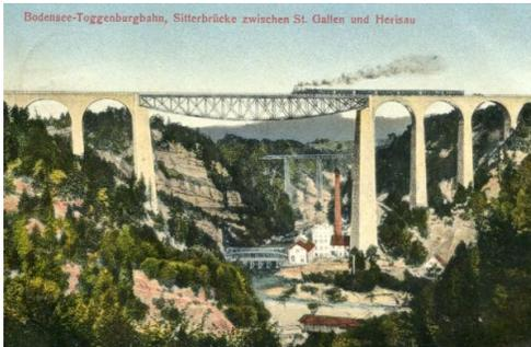
One of these viaducts, the Sitter Viaduct, is still today the highest rail viaduct in Switzerland towering over the Sitter Valley at 324 feet in height and over 1200 feet in length. In addition to the stone piers, the Sitter Viaduct also employed a distinctive steel truss framework known as a *Fischbauch* or "fish belly". A historic postcard (above) shows a B-T steam train going over the "fish belly".
