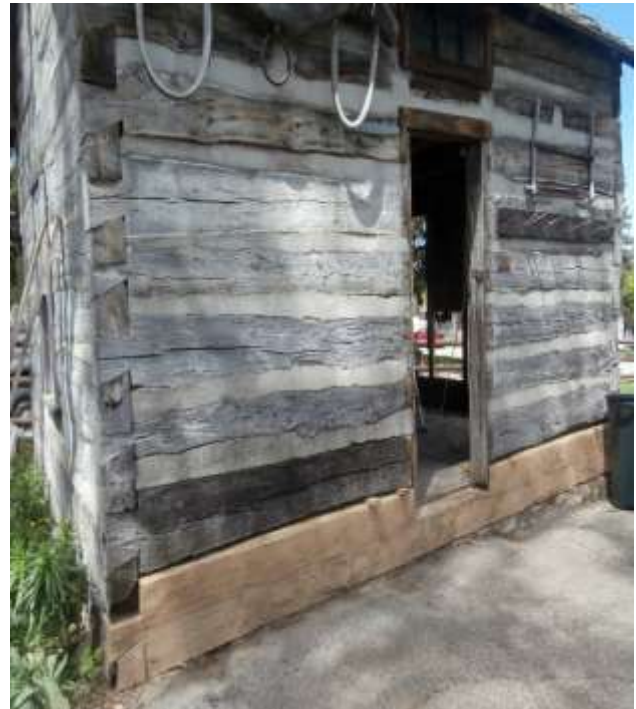
East side base log replacement
