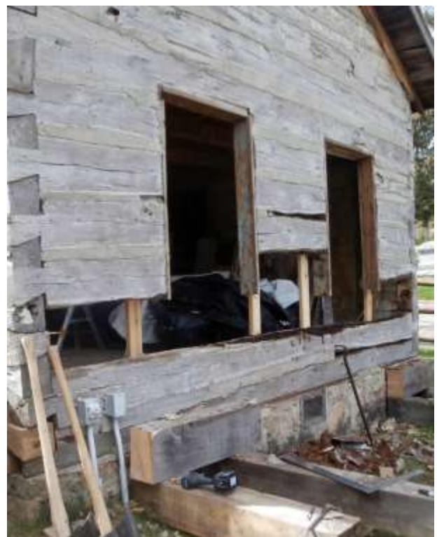
North side log removal prior to replacement
