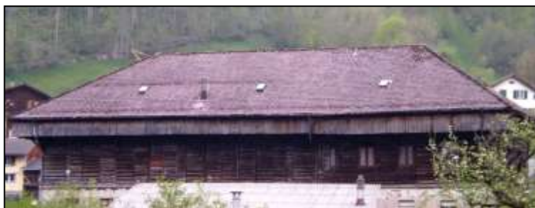
Hänggitürme [drying "towers"], once used for hanging newly dyed cloth in the open air under the eaves, still dot the Linth River valley. This one is in Ennetbühl. It was believed that open-air drying made the colors brighter.
